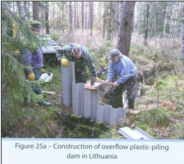
Figure 25a – Construction of overflow plastic-piling dam in Lithuania
